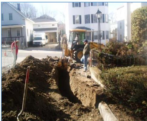
Workers from J. E. Amorello, Inc. install a new water line for our sprinkler system.
